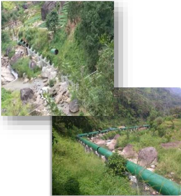
Move penstock pipes to the necessary locations using cables, considering the safety of the villagers and close residents
